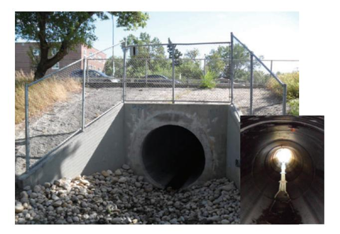
The City of Winnipeg decided in late 2010 to rehabilitate a large culvert under Portage Ave., a major highway through the city using Weholite high density polyethylene (HDPE) pipe. The Weholite culvert lining system is a no-dig solution for repairing culverts because it does not require excavation and does not require road closures or disruptions to traffic. In addition, no extensive equipment or training is necessary to install the Weholite pipe liner.
